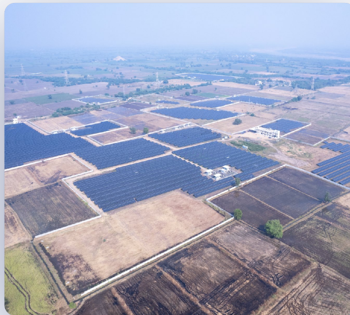
— ⚡ Utility Scale, Ground Mounted Solar Site, Gujarat
